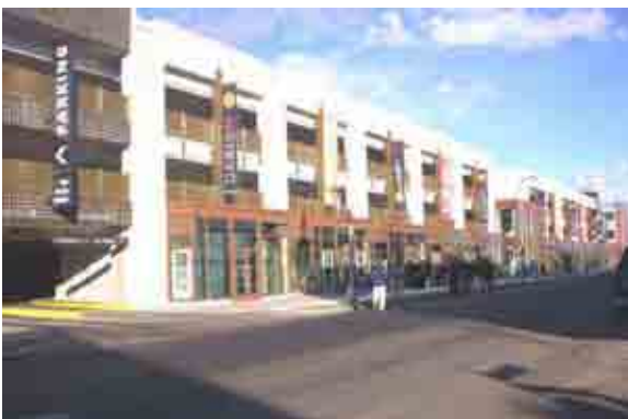
The parking garage is lined with display space on the first two floors along its entire street frontage.
