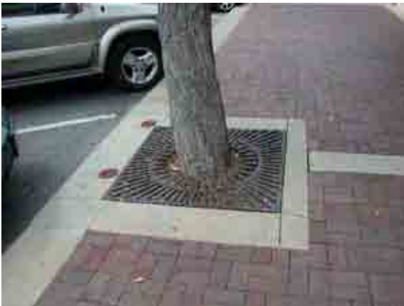
6.3.6 Tree Well. A tree well is an individual landscaped area surrounded by pavement.
