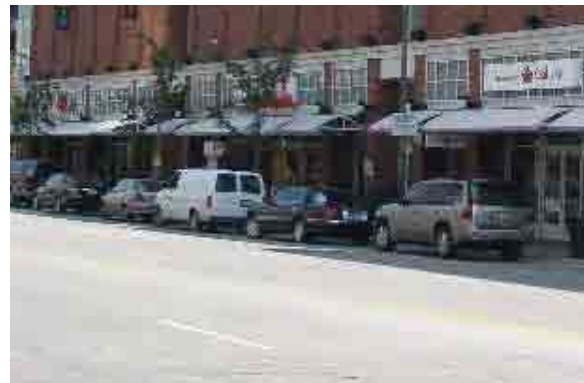
This parking garage is lined with retail space on the first floor along its entire street frontage.
