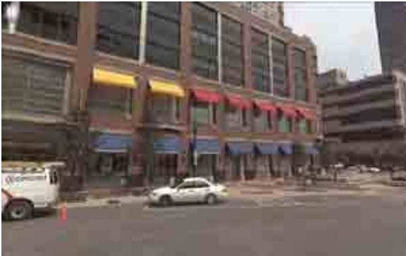
This parking garage is lined with retail and office space on the first two floors along its entire street frontage.
