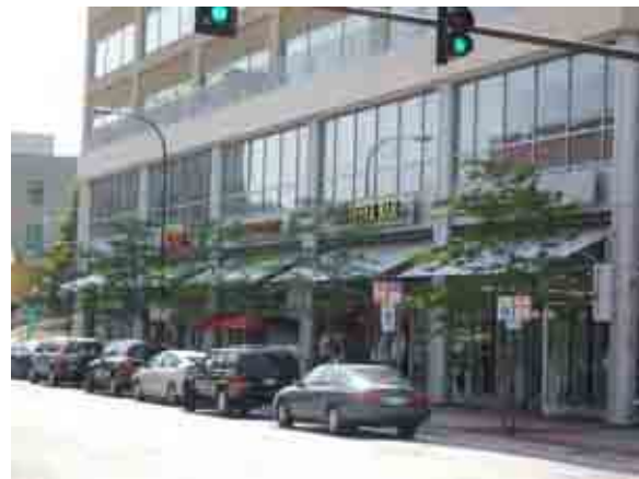
The parking garage is lined with retail and office space on the first two floors along its entire street frontage.
