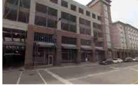
The parking garage is lined with retail space along the street frontage.
