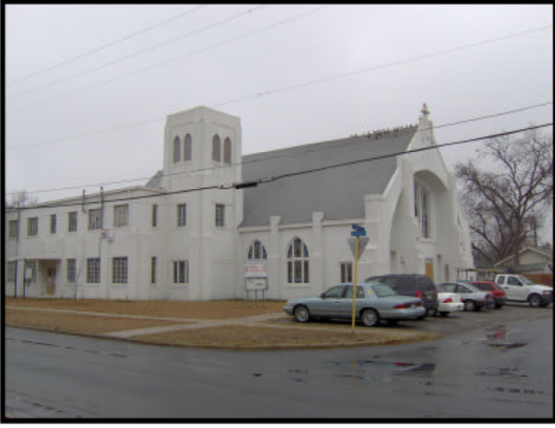
Palm Heights United Methodist Church Park and Marlay Street.
