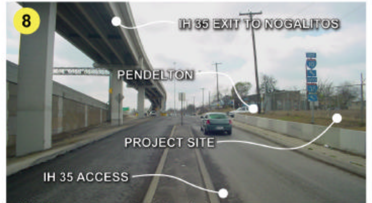
IH 35 access road at Pendelton
