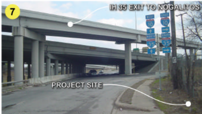
IH 35 access road to north and south ramps
