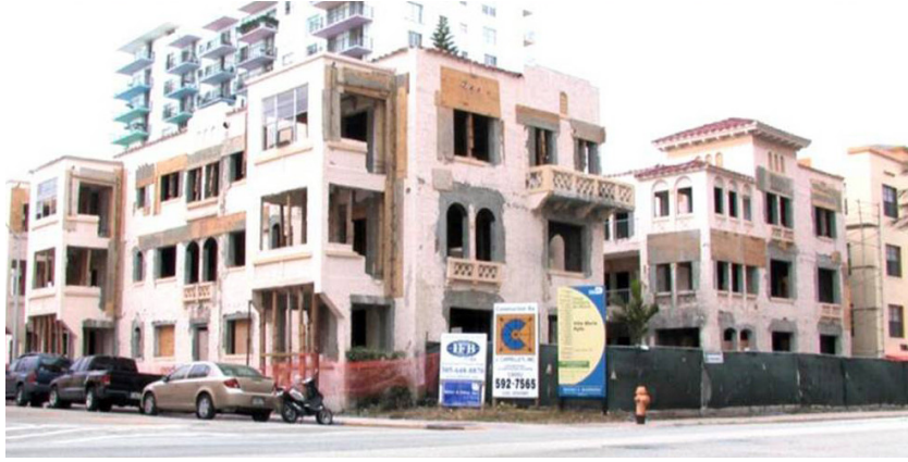
Prior to the renovations.
