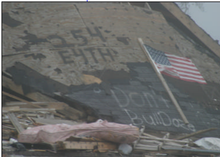
Damage from Hurricane Katrina
