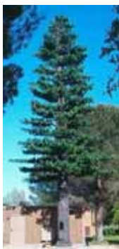
Monopine A cell tower "stealthed" as a pine tree
